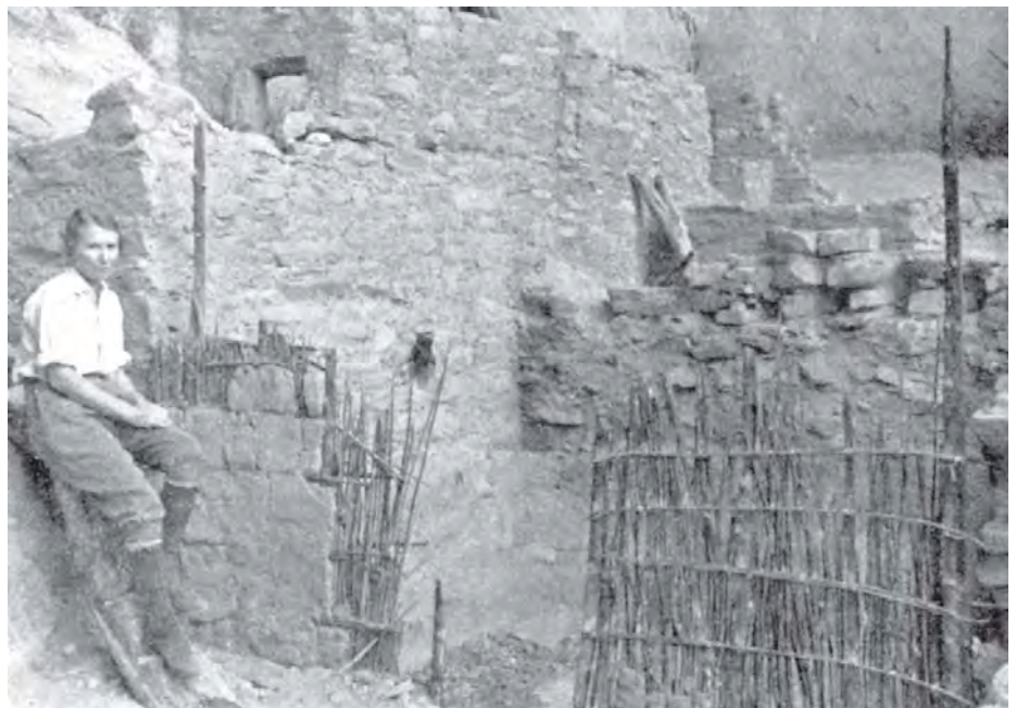
Figure 3: Early photograph showing wattle -and-daub wall construction at Anasazi Pueblo of Betatakin in Northern Arizona (adapted from McGregor 1977:328).
