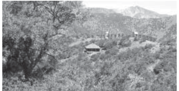
Figure 4: Stabilized structure, August 2001.
