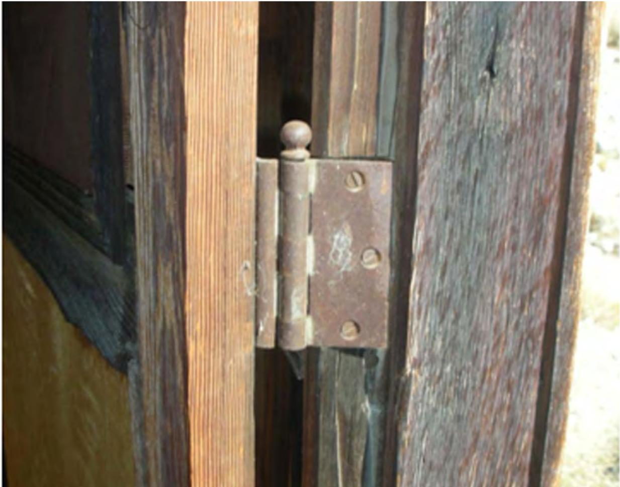
*Figure 6. Door repair showing planed surface on door edge, replacement panel (at left) and reuse of original ball top hinge.*
