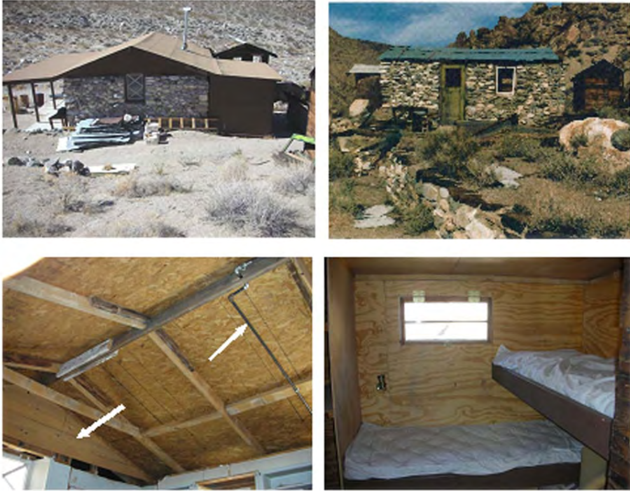
Figure 8. (upper left) Osborne Cabin as it currently appears, side view toward northwest showing porch and shed additions; (upper right) southwest aspect (front) and outbuildings ca. 1997, view northeast (Photograph: BLM); (lower left) replacement rafters and sub-roof, with original ridge board still in place. Gas pipe and panel infill of gable space are also shown (at arrows); (lower right) detail of north wall of sleeping room taken from passage from original cabin.
