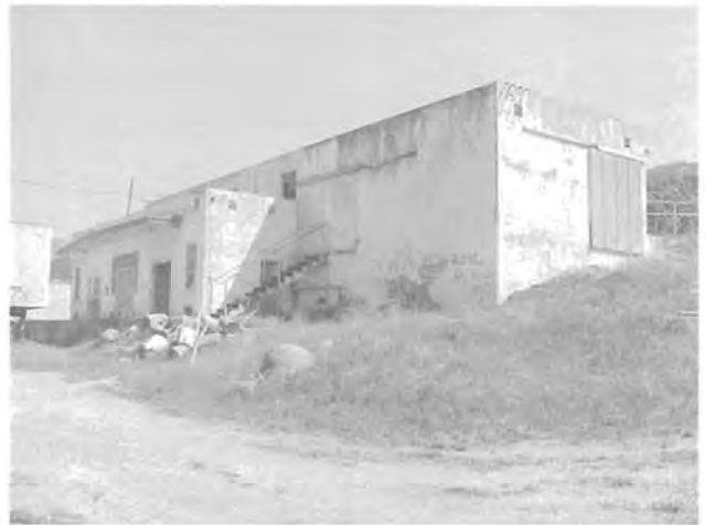
Figure 8. The Earl Bishop Dairy, oblique view.
