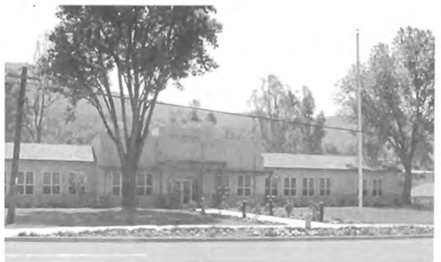
Figure 12. The San Pasqual Academy after renovation in 2001.
