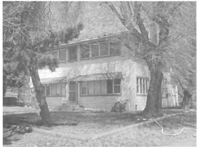
Figure 2. The Olds residence, oblique view.
