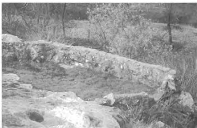
Figure 18. Stone and mud-mortared catch-basin from the late 18 th or early 19 th century.
