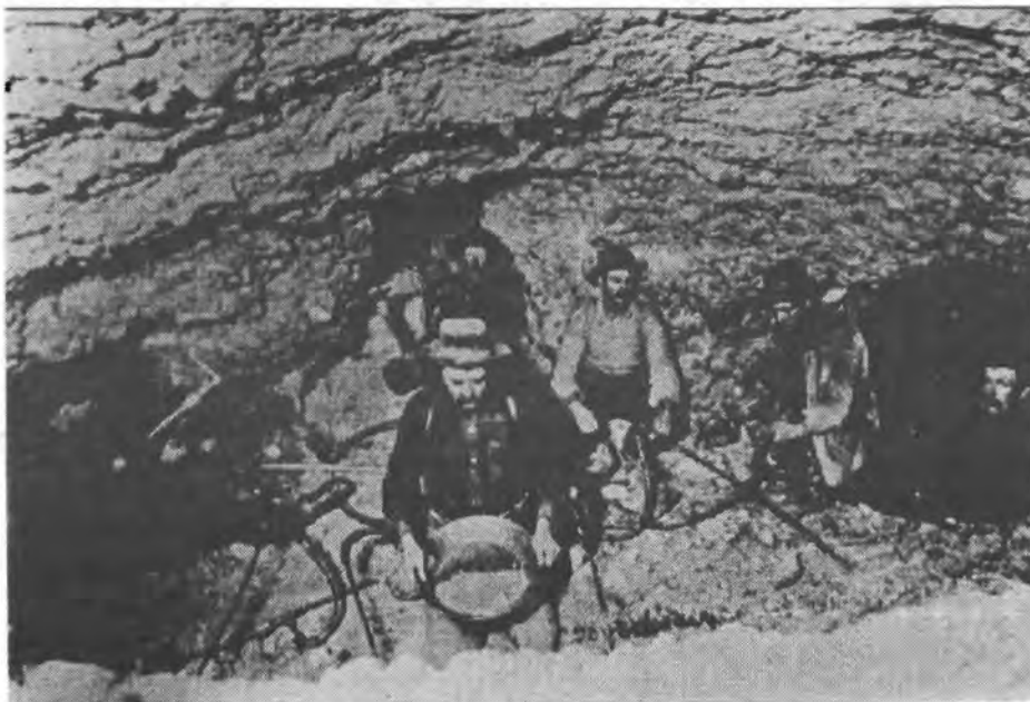
Figure 10. Drift mining works placer deposits by underground methods.
