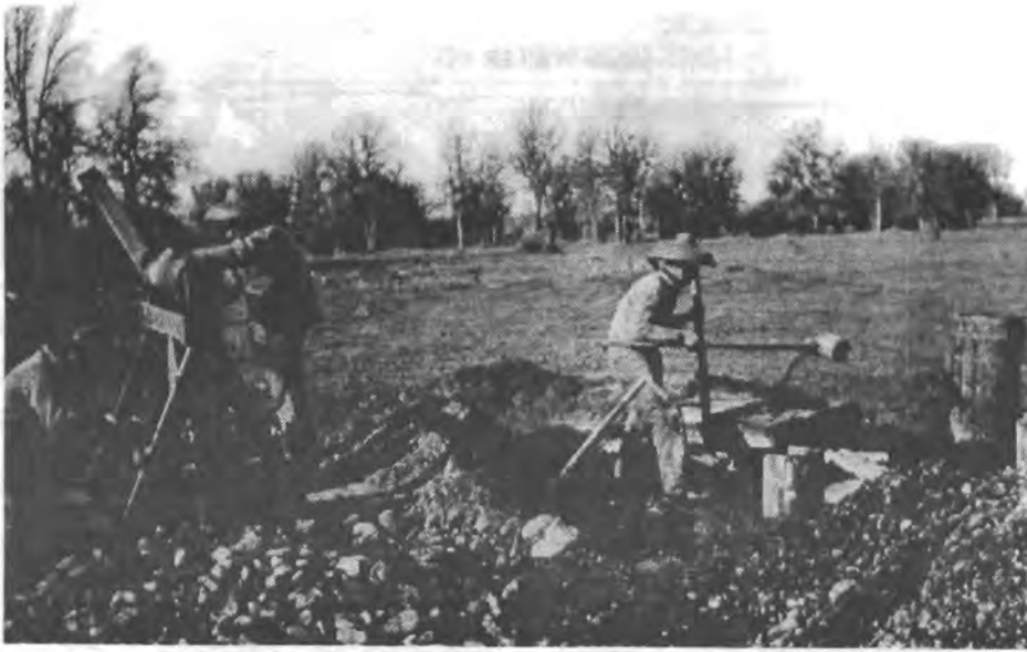
Figure 9. Chinese miners ca. 1900. Drift mines are worked through vertical shafts sunk to bedrock. From the bottom of the shaft, drifts are run along the bedrock and the pay gravel is brought to the surface by a windlass where it is washed in rockers or sluices.
