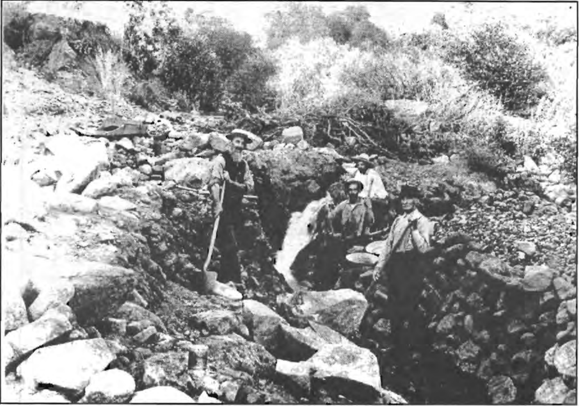
Figure 12. Ground sluicing in El Dorado County
