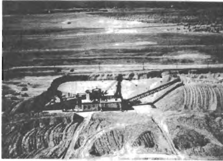
Figure 17. Bucket-line dredge, Natoma No. 6 working approximately one mile south of White Rock Road and ½ mile east of Sunrise Boulevard, Folsom, September 7, 1959.
